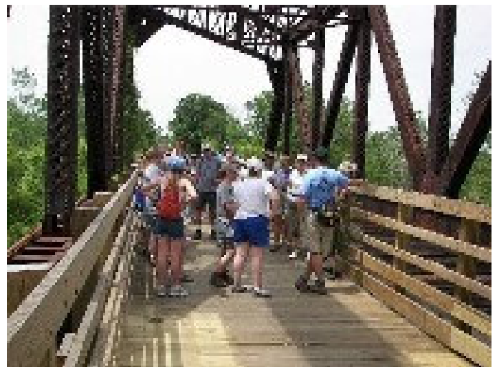
The recently redecked trestle on the Lehigh Trail.
